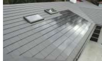
Solar Roof Inserts
