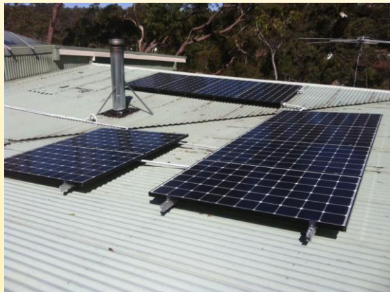
5kW of LG 315 Flat on roof
